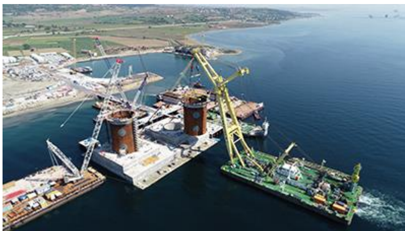
Steel shaft erection on the Asian side of the crossing
