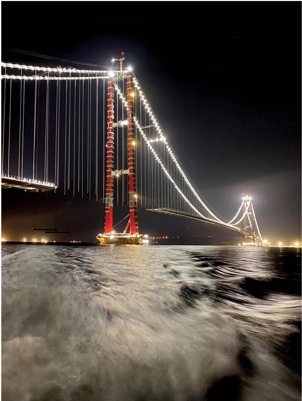
Crews worked in a climate that is often rainy and windy, with strong currents. Asian Hercules III, a 5,000-tonne floating crane (bottom left) from Singapore, erected deck segments in carefully planned windows of time when the wind was not too severe. Photo courtesy of DLSY JV
