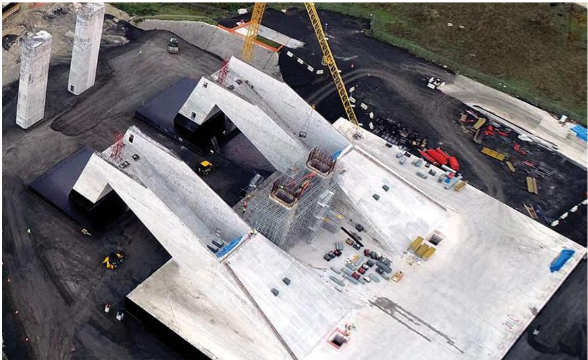
Anchorage weigh 160 tonnes and were cast in 2-m layers, each with six segments. Photos courtesy of DLSY JV
