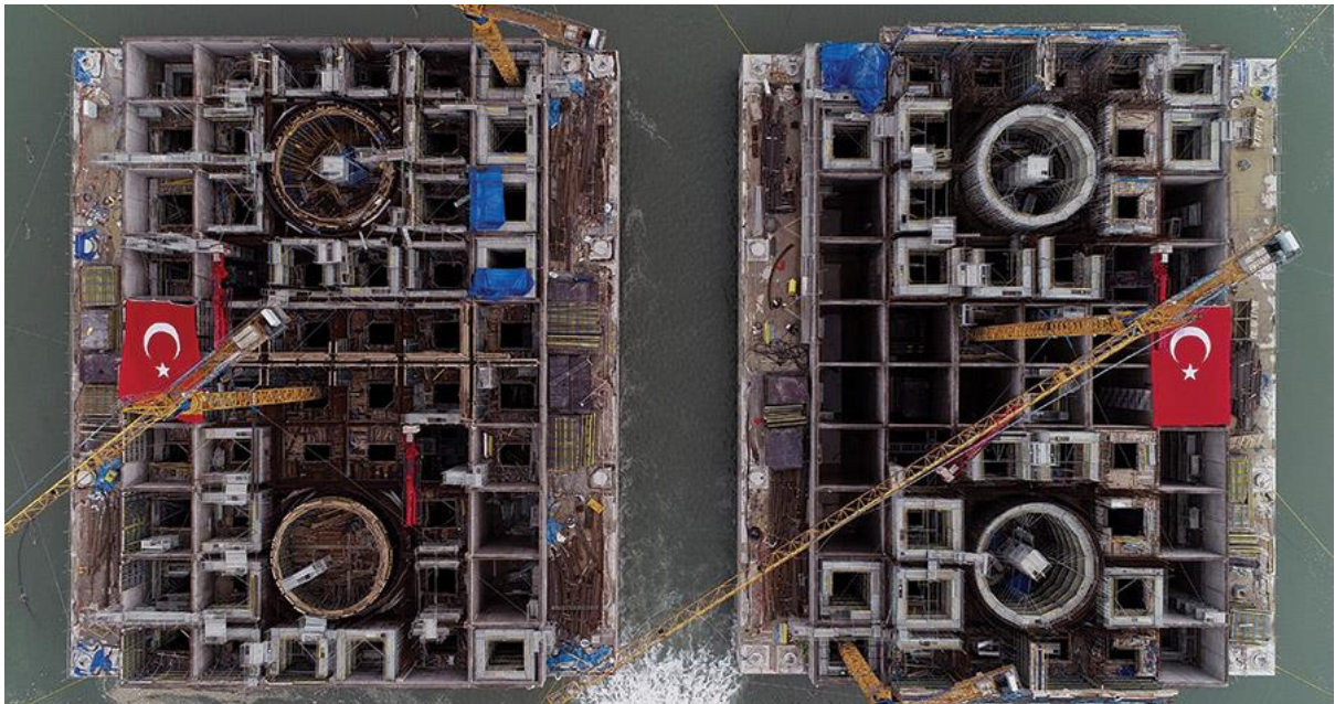
A dry and wet dock were built to facilitate placement of caissons that form the massive tower footings. Photos courtesy of DLSY JV
